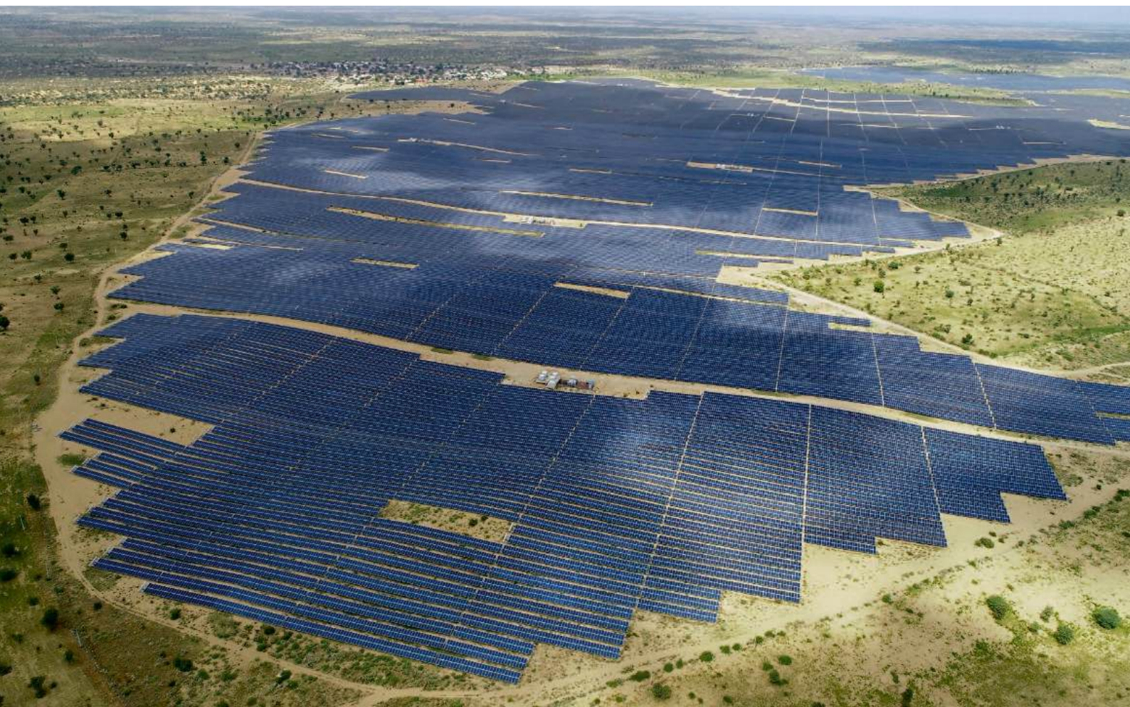
Solar Plant, Bikaner
